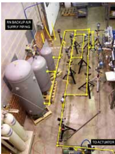
Figure 3. Overall test set up, highlighting both the 1/2" and 3/4" air supply circuits
