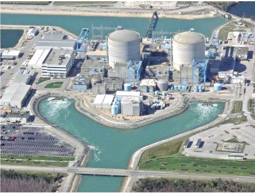
St. Lucie Nuclear Power Station, Florida, USA
