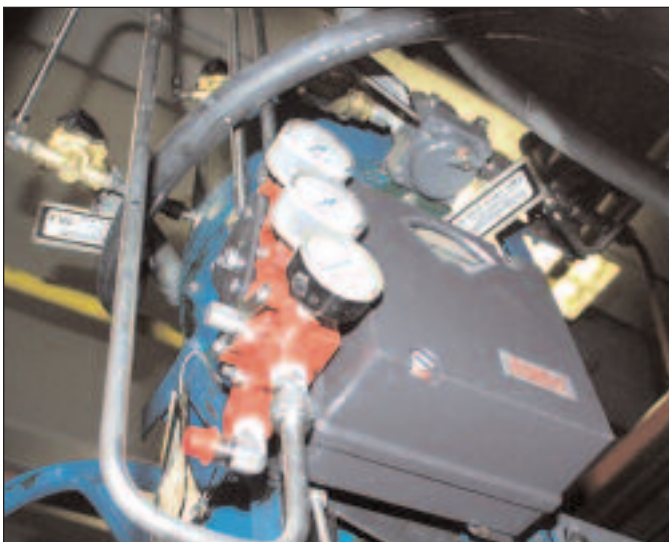
Figure 2. Original installation with spool valve positioner
