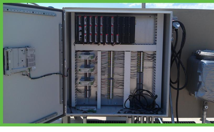
A ROC800-Series RTU can be appropriately sized for almost any application. The ROC809 and ROC809L provide nine slots for I/O and communications modules. The ROC827 and ROC827L models offer 3, 9, 15, 21, or 27 slots using optional expansion module racks.
