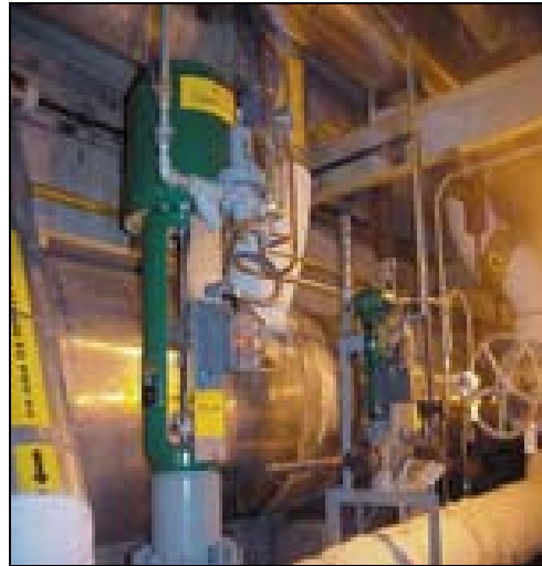
Figure 2: 12" TBX Steam Conditioning Valve
