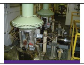
BEFORE —The original feedwater recirculation/startup valve assemblies included problematic positioners, exhausts, and solenoids. The unreliable combination of instruments required manual control during startup and resulted in costly delays or plant trips.
