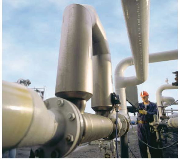
Coriolis meters are accurate and reliable. Because there are no moving parts, maintenance is reduced to a minimum.
