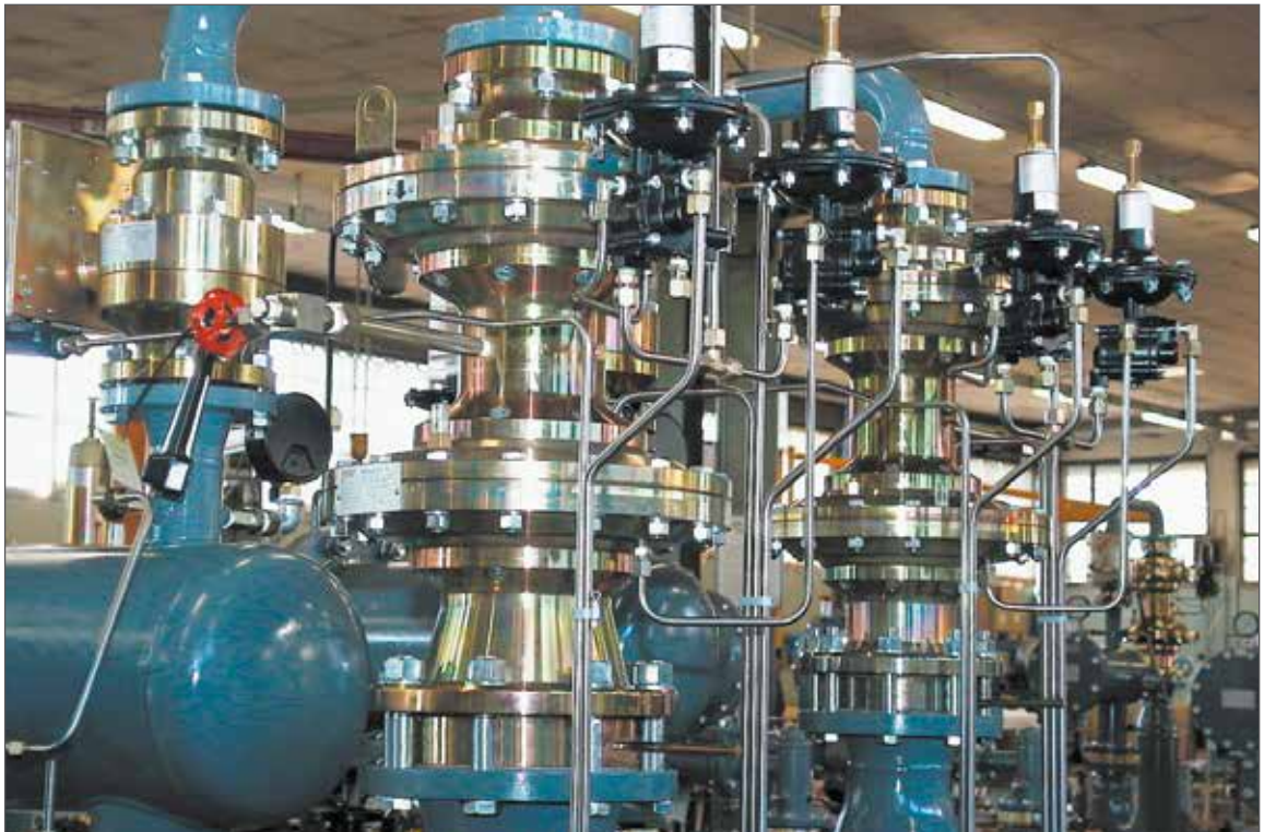
Regulation Skid Detail
